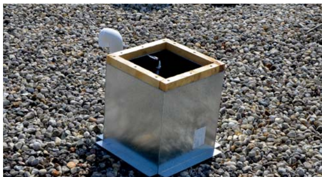
New curbs are being installed prior to the arrival of the new insulation and membrane. The curb will have the base flashing installed and the interior sealed and waterproofed prior to membrane installation.
