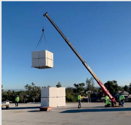
Crews from Multi-Pro Roof Solutions re-covered the existing built-up roof system with the new TPO system.
