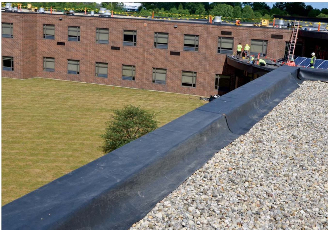
The roof edge coping is completely flashed and measured for the new sheet metal fabrication. The base flashing is left loose on the interior side and will be integrated into the new roof cover.
