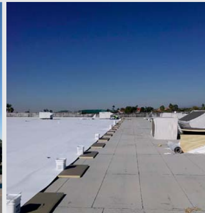
Crews from Multi-Pro Roof Solutions re-covered the existing built-up roof system with the new TPO system.
