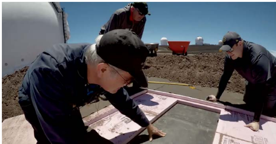
The existing EPDM roof system is inspected prior to the PV installation. The inspection and non-destructive testing confirmed the more than thirty-year-old membrane was in excellent condition.
