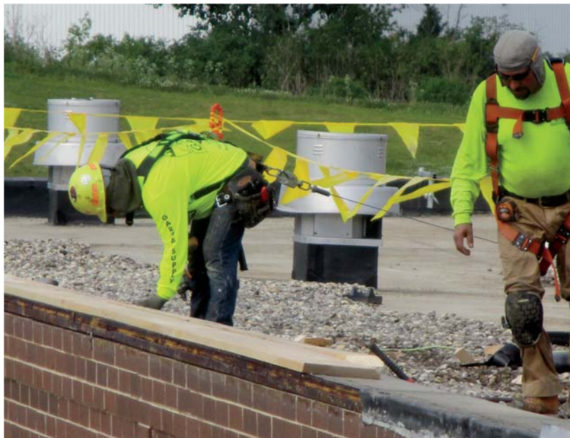
The contractor removed the roof edge coping, raised the roof edge and then installed the new base flashing that will be integrated into the new roof cover.
