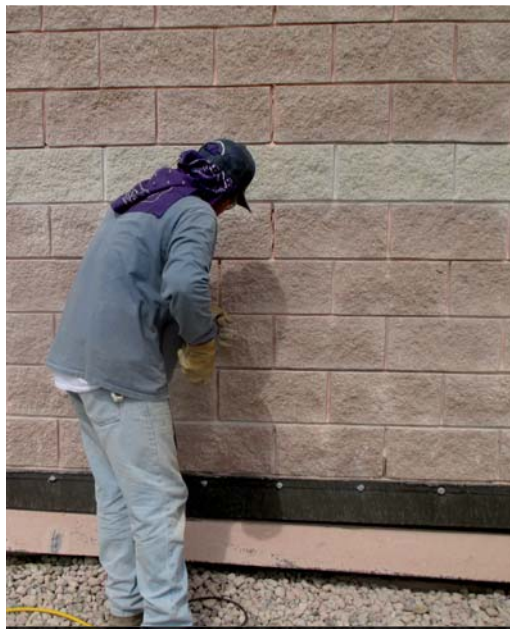
Having masonry work completed prior to the new roofing installation prevents potential damage to the new roof.
