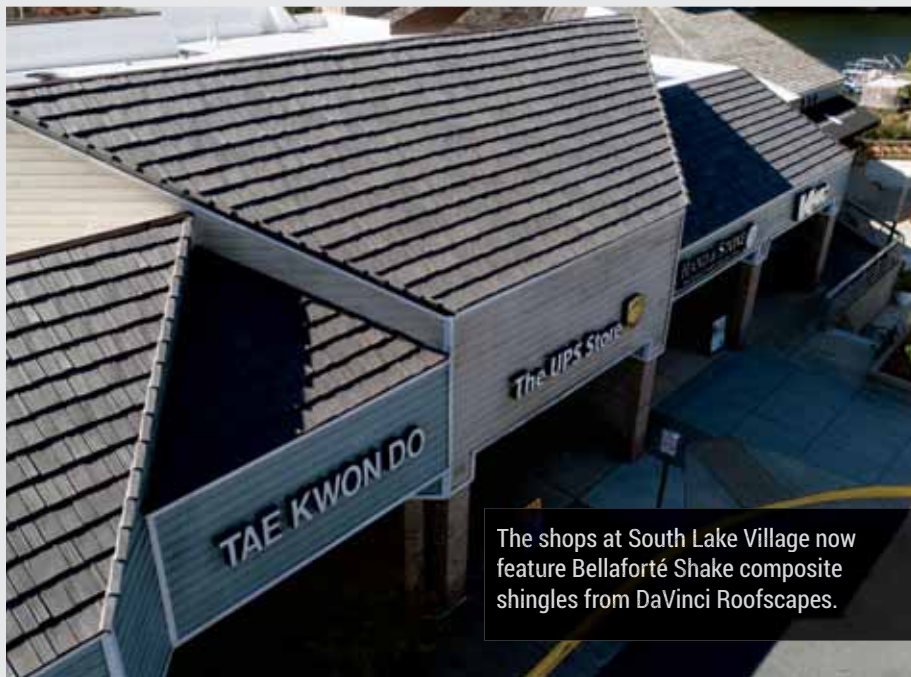
The roof replacement project at South Lake Village Shopping Center included a new TPO roof system on the low-slope section and synthetic shake on the steep-slope sections.
