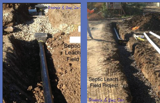
Installation of new leach field.
