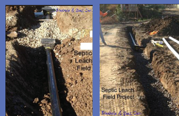
Installation of new leach field.
