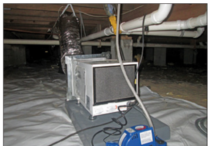
This is one of two units in a very large crawlspace to keep dry air circulating everywhere.
