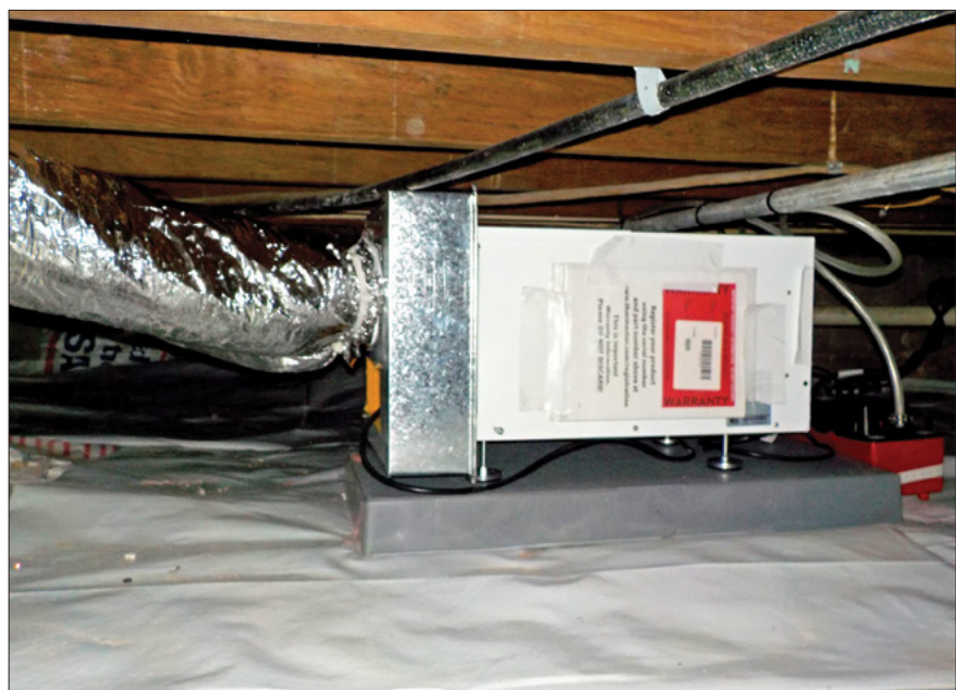
A dehumidifier system keeps crawlspace dry.
