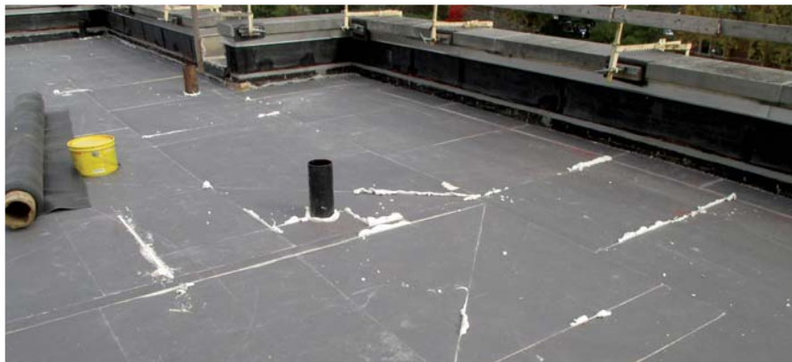
The connection between the membrane and the perimeter of the building requires special attention. There should be no voids in the insulation at the perimeter.
