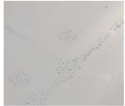
Photo 5 Heat loss through the insulation and the mechanical fasteners was so great that it melted the snow, which later froze again.
