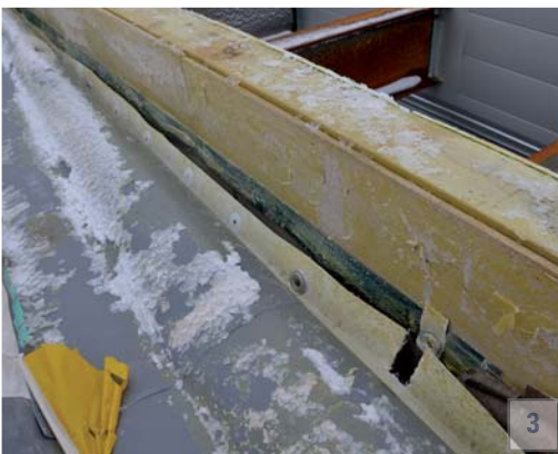
Photo 3 All the base anchor screws pulled out of the substrate except one that was into the stud, which just tore away when the rest of the membrane lifted.
