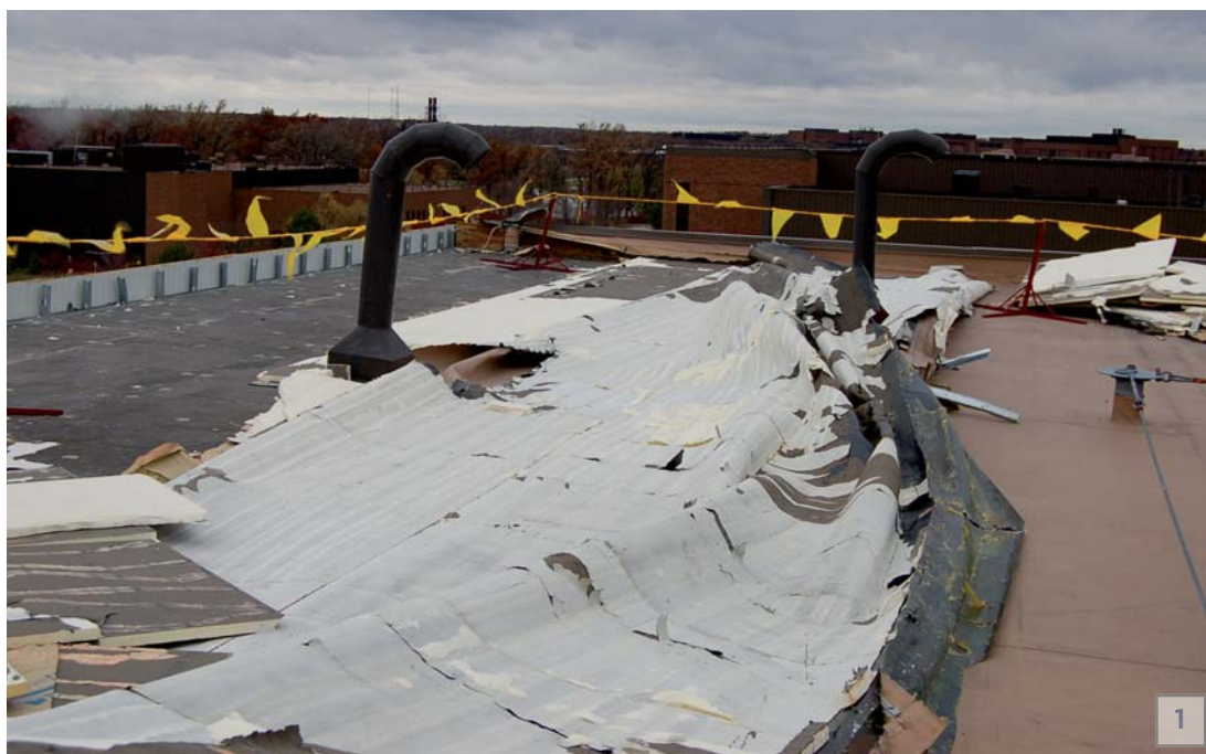
Photo 1 With a stud wall parapet, inappropriate wall substrate and base anchor screws into a material with low pull-out resistance, this roof blew off in what would be considered moderate winds.
