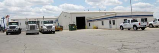
24,720 SF Available, 1.60 AC Hard Surfaced, Fenced-In Outdoor Area
