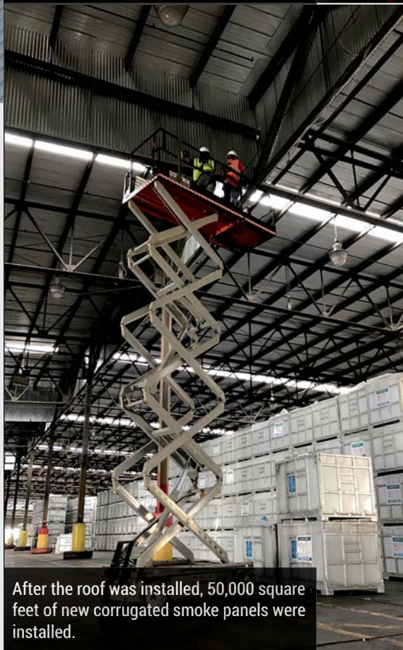
Crew members on lifts reinforced the existing steel structure before the new roof was installed.
