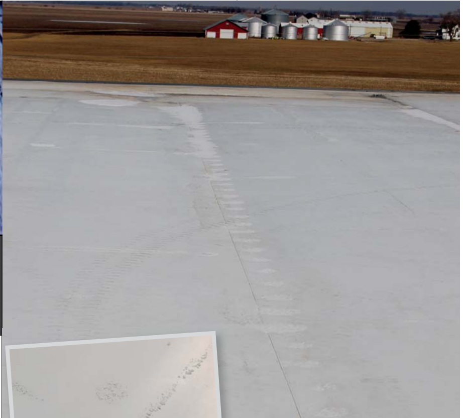
PHOTO 2. When a light dusting of snow blew off this 2 million-square-foot facility in central Illinois, every single mechanical fastener and insulation joint could be identified by the ice visible at their locations. This roof needed to be replaced due to condensation issues several years after installation at a cost of more than $10 million.
