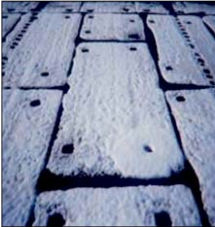
PHOTO 1. Conditions such as this, in which the fastener plates melt the snow, visually demonstrate the heat loss that is a known entity to roof installers and knowledgeable roofing professionals.
