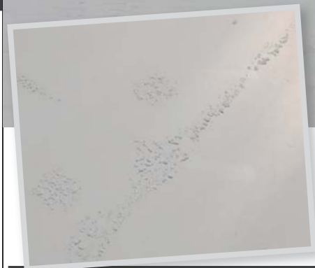
PHOTO 3. This is close-up of the roof shown in Photo 2. Heat loss through the screws and fastener plates and through joints in the single layer of insulation melted the snow. The water froze when the temperatures dropped and the ice was revealed when a light wind pillowed the membrane and the remaining snow blew away.
