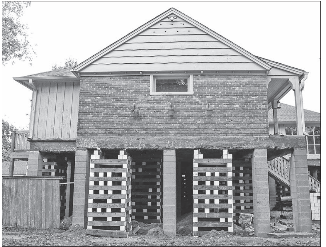
A home in the Meyerland neighborhood of Houston is in the process of being raised by Arkitekture Development. ELIZABETH CONLEY/HOUSTON CHRONICLE VIA AP
