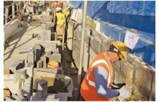
**Top to bottom:** 60 feet of rock had to be blasted and removed to prepare the site, requiring nearly 2 years and 25,000 truckloads of rock removal. Construction of the 287,000 sq. ft. building began once the site was prepared. The granite facade of 167, 901 bricks was installed by masons on site.
