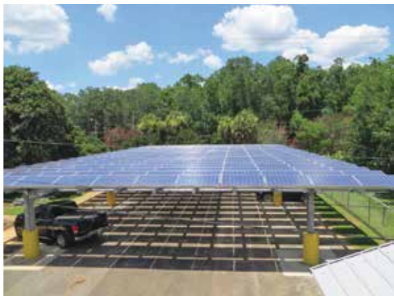
▲ Leon County's net-zero building is powered by a 60-kilowatt solar array that doubles as shaded parking.
