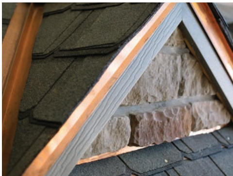
A small dormer shows examples of copper flashing and construction options in the showroom of Dale's Roofing.
