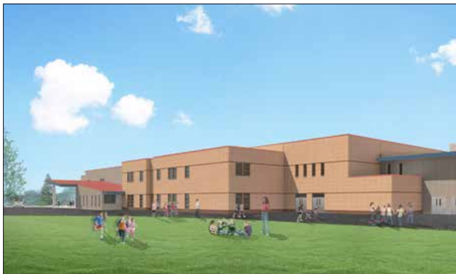
Kraus-Anderson was recently awarded a contract to manage a $93.9 million project that includes this expansion of Hudson High School, 1501 Vine St. in Hudson, Wisconsin.
