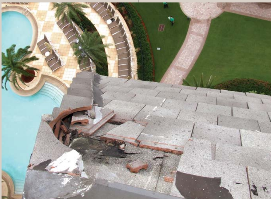
A lightning strike on a hotel on Marco Island, Fla., shattered concrete roof tiles and created a hazard to people and facilities 10 stories below. A fire could have resulted if the building had a wood frame instead of a non-combustible structure.
