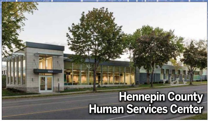
Knutson Construction cut new holes for more than three dozen 12-foot-high windows as part of converting a former printing facility into a Hennepin County Human Services Center.
