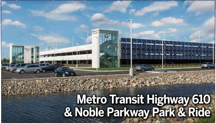
Metro Transit's environmental focus for the park & ride facility in Brooklyn Park extends to the outside, where low-level water filtration areas and ponding cleanse rainwater runoff.
