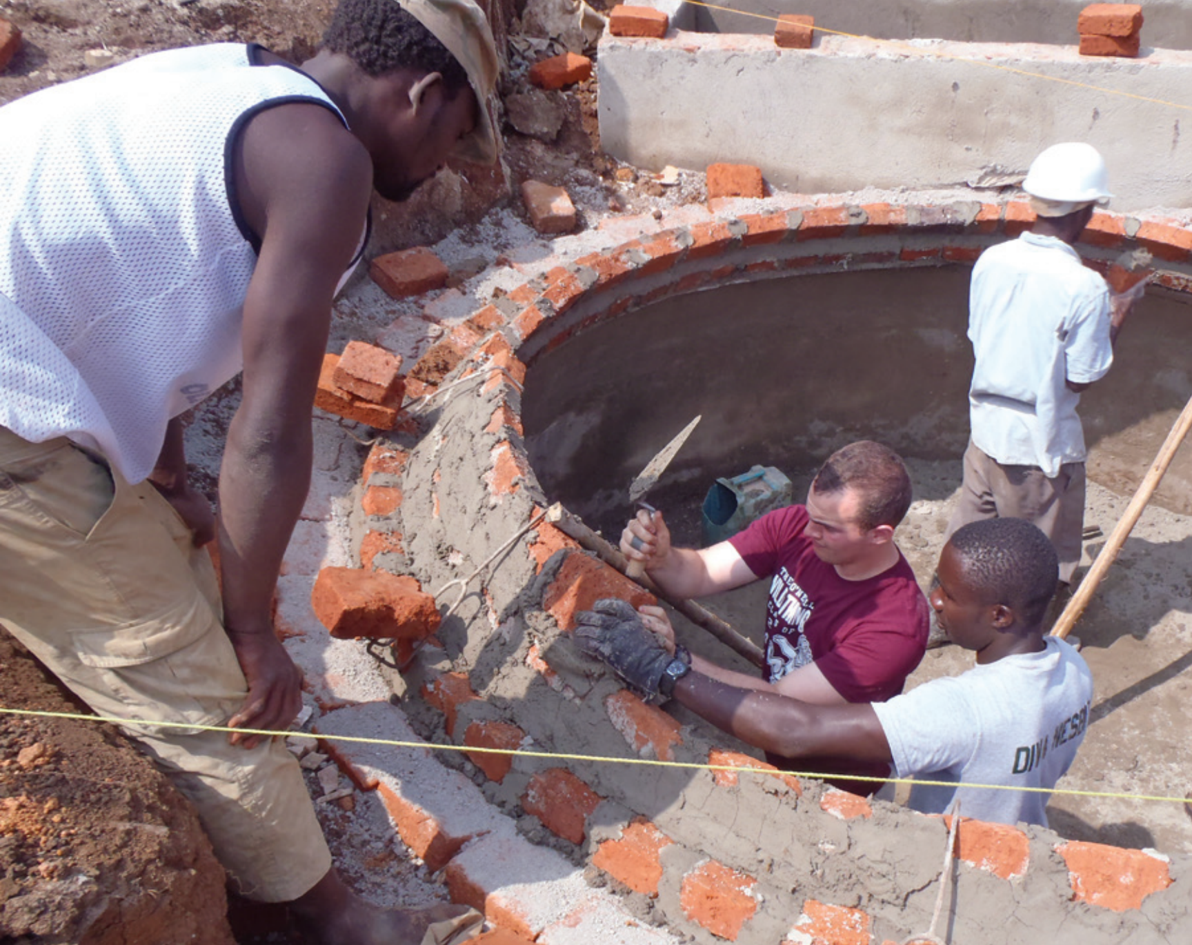
CDT Pat Bastianelli '15 constructs the dome of a biogas system during a 2013 AIAD in Uganda, Africa.
