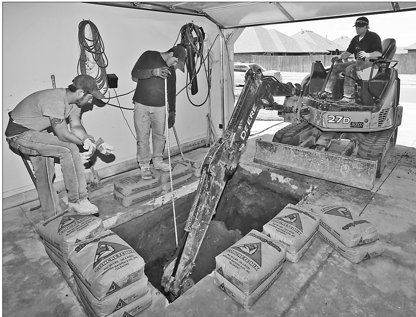
Thunderground Storm Shelters’ Dustin Wagner, left, and Jacob Ortiz, center, assist as Jim Hohnsbehn digs a hole for a storm shelter in the garage at a residence in Oklahoma City. AP PHOTO/SUE OGRICKI
