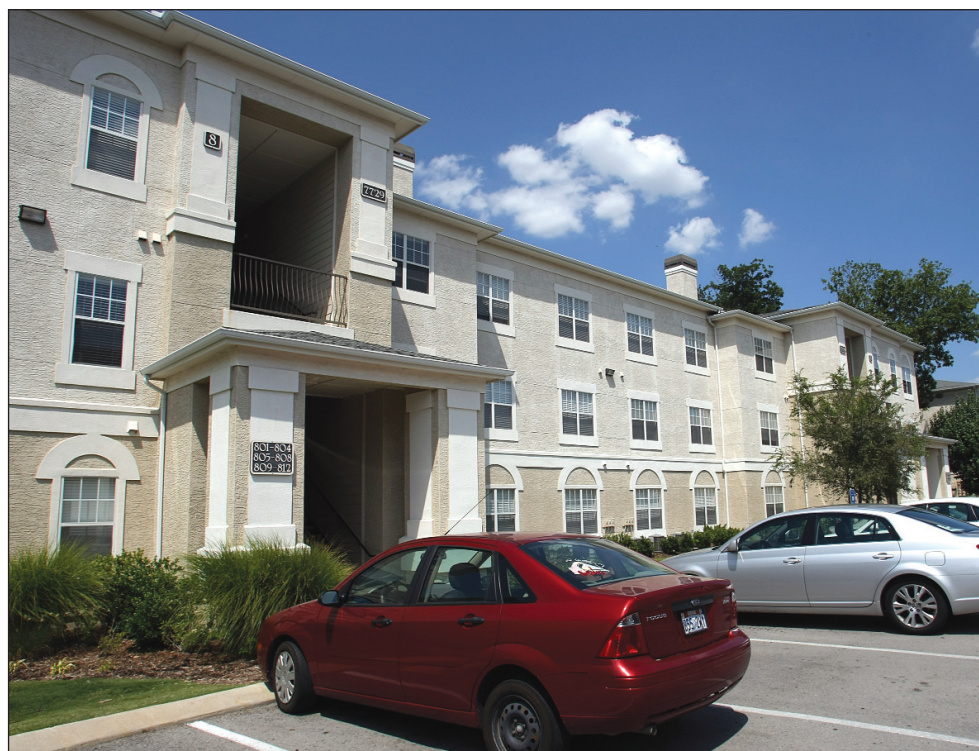
The 294-unit Estancia Apartments at 7705 S. Mingo in Tulsa sold to Steadfast Asset Holding Inc. for $27.9 million. PHOTO BY RIP STELL
