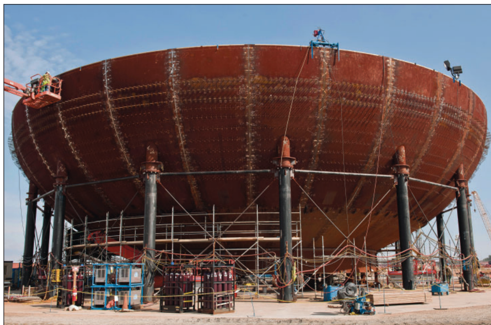
Construction crews work on assembling a containment vessel at Plant Vogtle in Georgia; the two additional reactors being built are the first new reactors approved by the Nuclear Regulatory Commission in 30 years.
