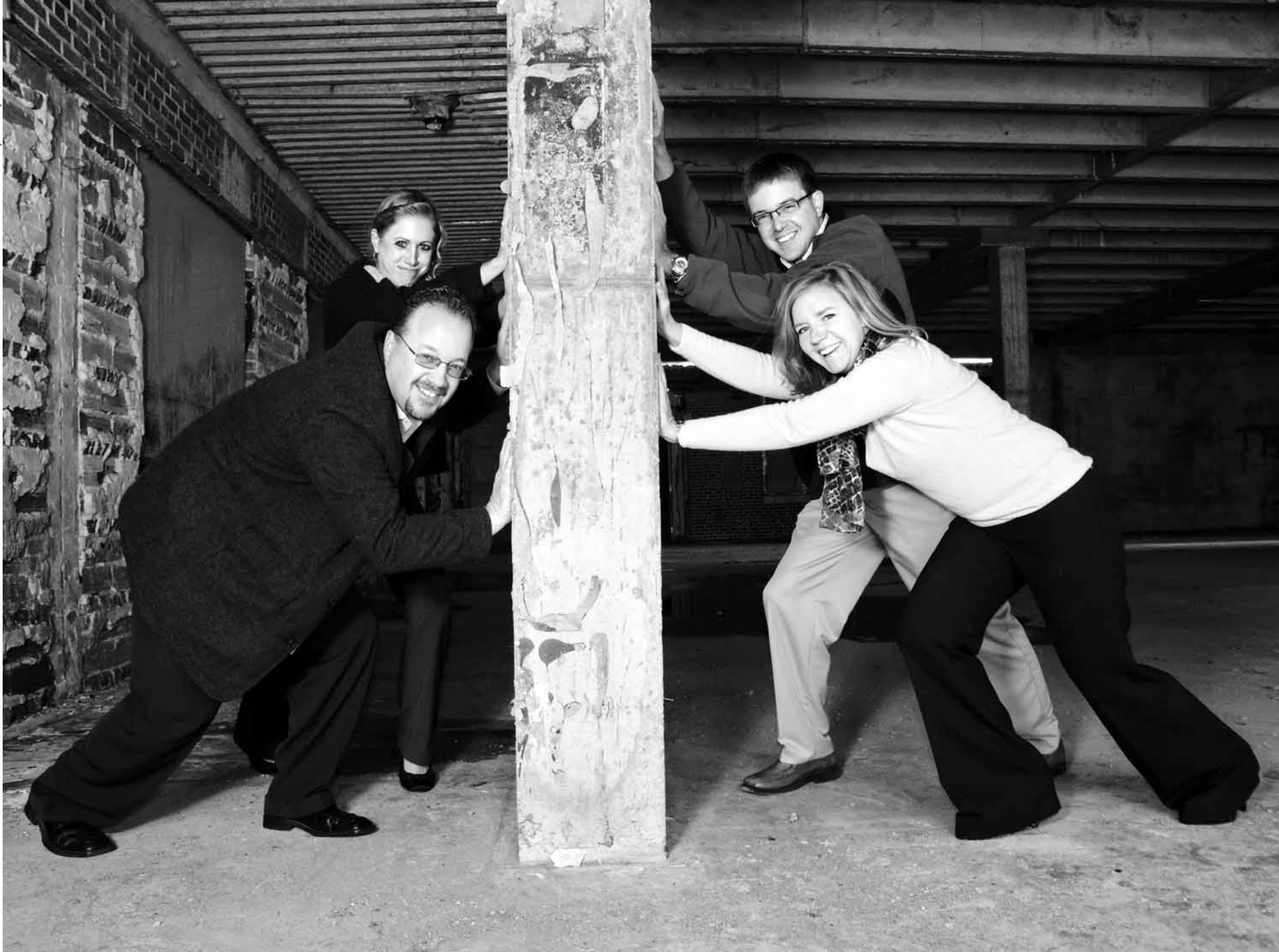
Clockwise from bottom left: McDonnel Group employees Bill McDonnel and Deanna LaFrance play a reverse tug-of-war with Andy Rredmon and Tricia LaFleur on a concrete column at the St. Margaret's Daughters Home, which the firm is renovating.
